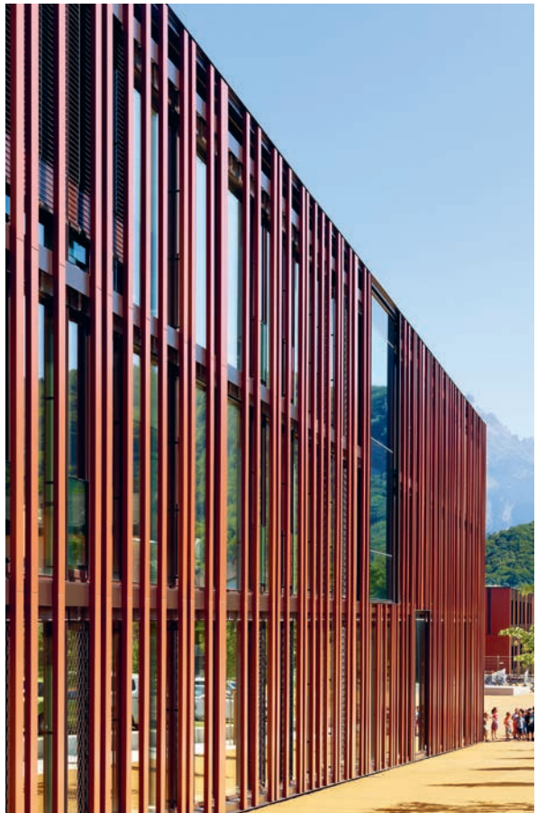
School building, Collombey-Muraz
